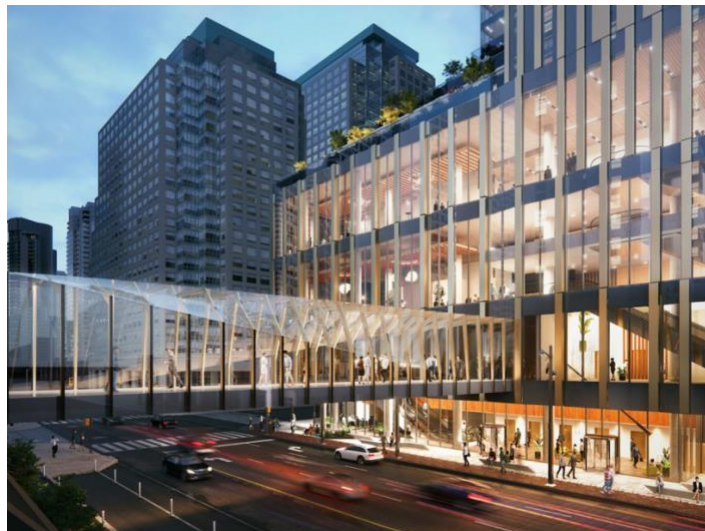
New tower coming to 11 Bay St. with expanded Queens Quay Station below.
