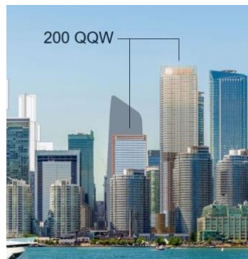
200 Queens Quay W. Plans show 71-storey tower with 1,482 new condos at Simcoe St.
